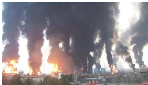
Figure 14. Massive fire in IOCL tank terminal [6]
