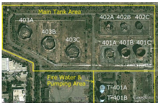
Figure 13. Main Tank Area of IOCL tank terminal (from Google Earth)
