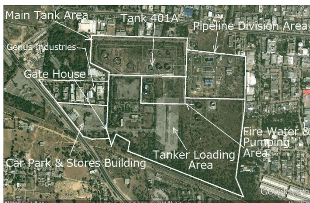
Figure 12. Layout of IOCL tank Terminal (from Google Earth)
