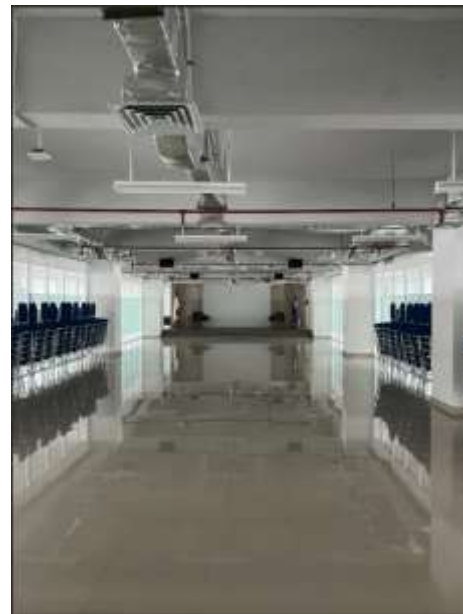
Figure 4. Interior condition of student lounge
