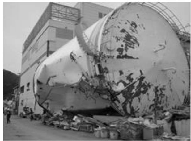
Figure 17. AST moved to higher ground and overturned by the tsunami at the 2011 Great East Japan Earthquake (Courtesy of National Research Institute of Fire and Disaster, Japan)
