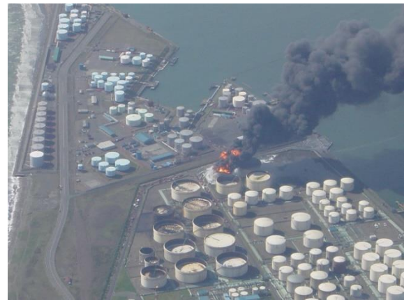
Figure 14. Aerial photo of full surface fire in a 30,000m 3 naphtha storage tank in Tomakomai at the 2003 Hokkaido Earthquake (Courtesy of National Research Institute of Fire and Disaster, Japan)
