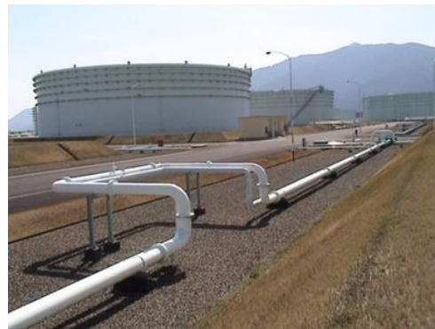
Figure 1. Aboveground storage tank (AST)
