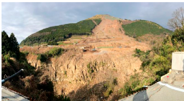
Fig. 5. Wide-angle view of the Great Aso Landslide that destroyed the bridge, whose remnant abutment is visible in the foreground of the photo (Kayen et al. 2016).
