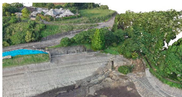
Fig. 6. Three-dimensional (3D) model of the spillway generated by UAV data (Kayen et al. 2016).
